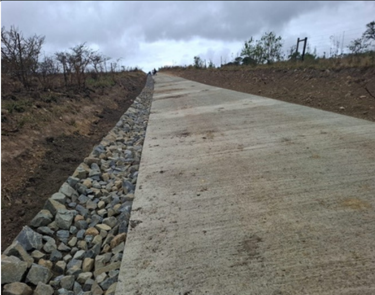
NGXINGXOLO/ KWENXURHA ACCESS ROAD
