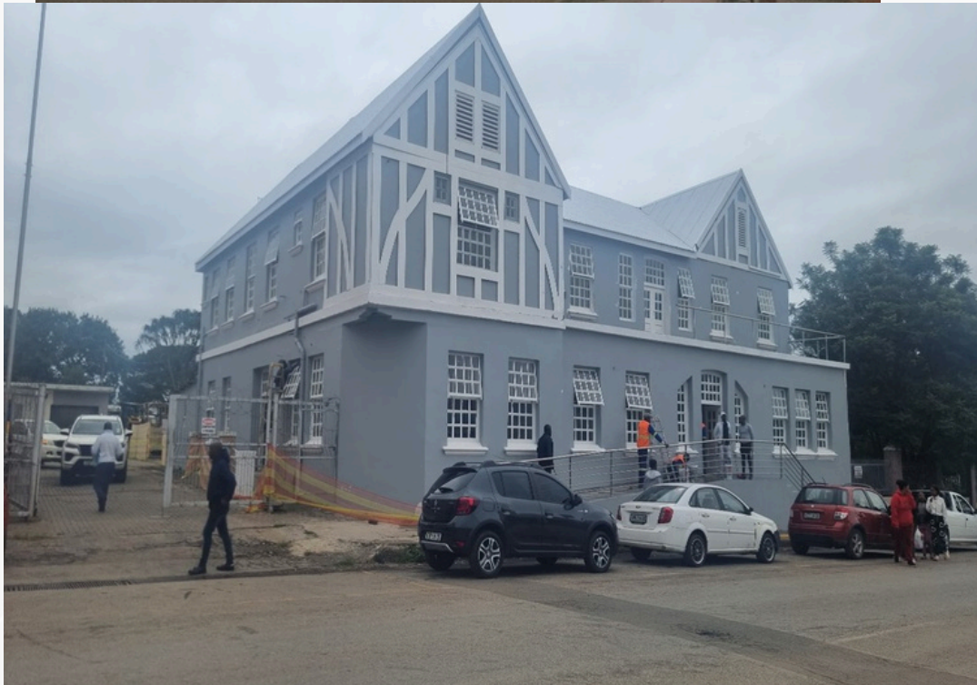
THE NEWLY RENOVATED MUNICIPAL BUILDING
