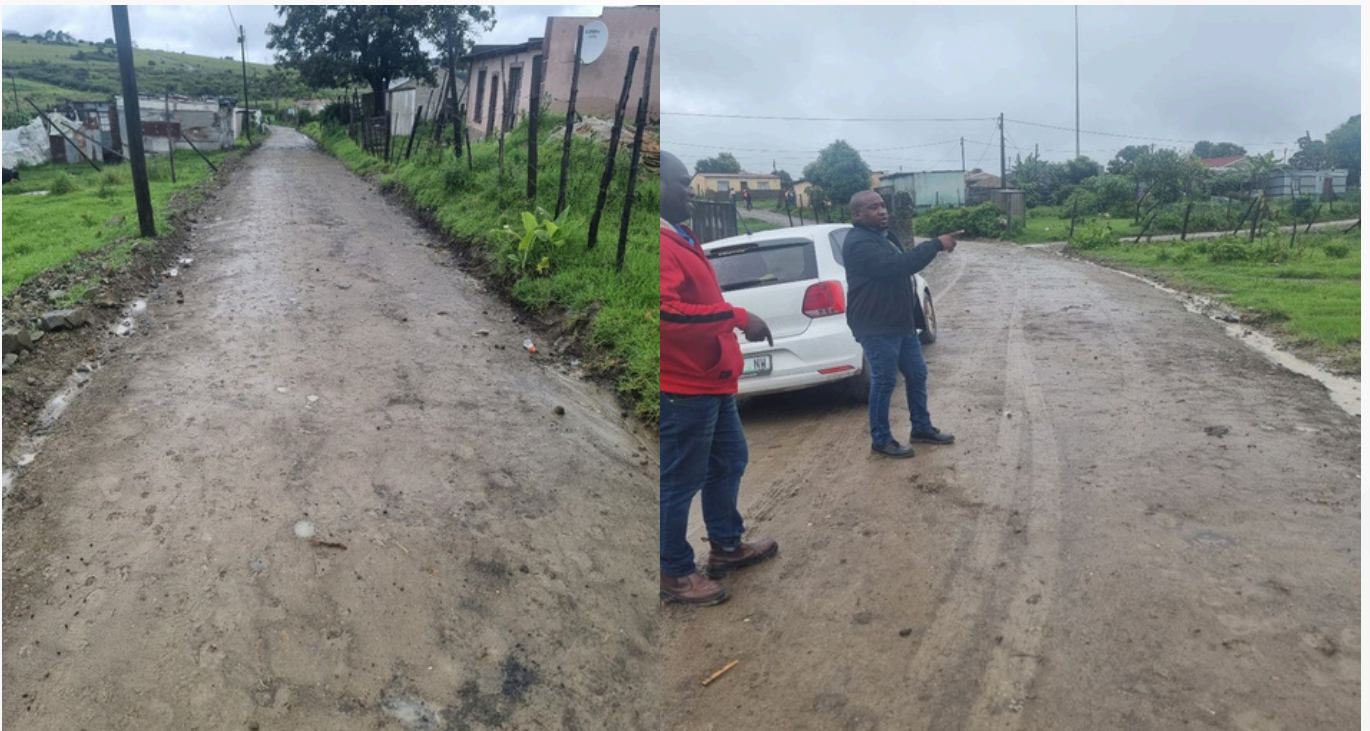
CONSTRUCTION OF OLD LOCATION
