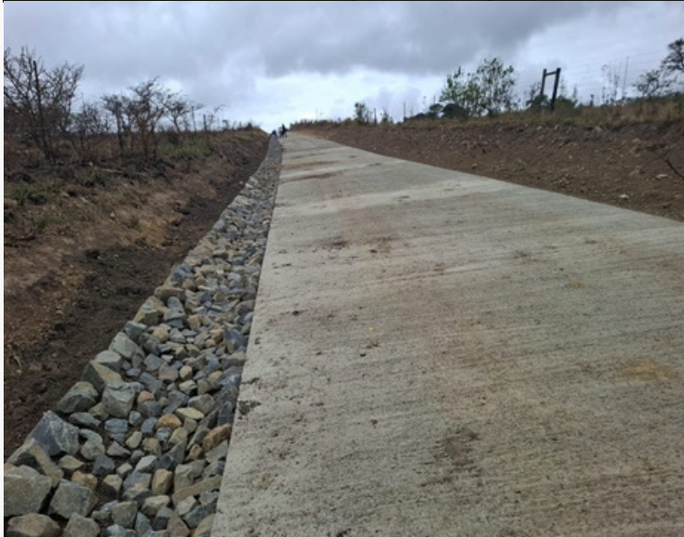
NGXINGXOLO/ KWENXURHA ACCESS ROAD
