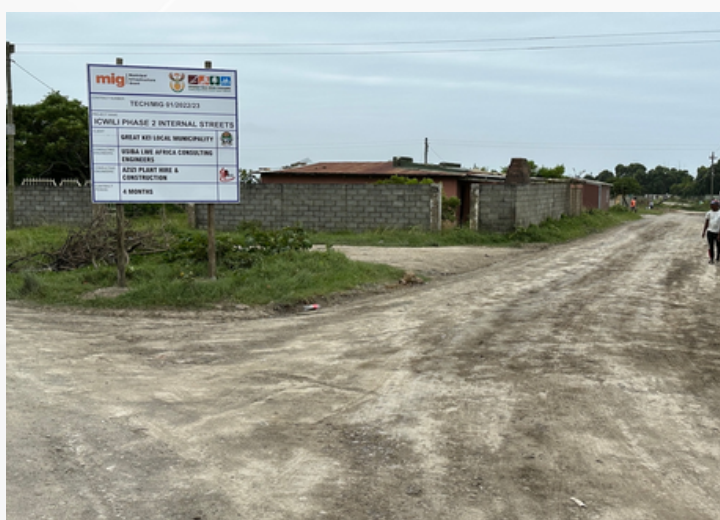
ICWILI INTERNAL STREETS PHASE 2 – WARD 5
